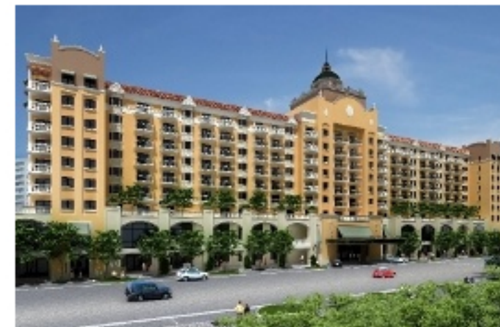
The residential component of The Palace at Coral Gables is a beautiful Mediterranean Palazzo-styled, nine-story tower with 243 luxury residences inspired by the world-renowned Four Seasons George V Hotel in Paris.
